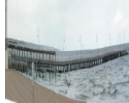
Kerferd Road Pier Port Melbourne March 2003 003
