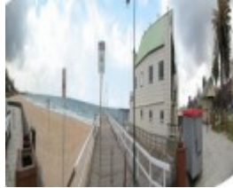
Kerferd Road Pier Port Melbourne March 2003 002
